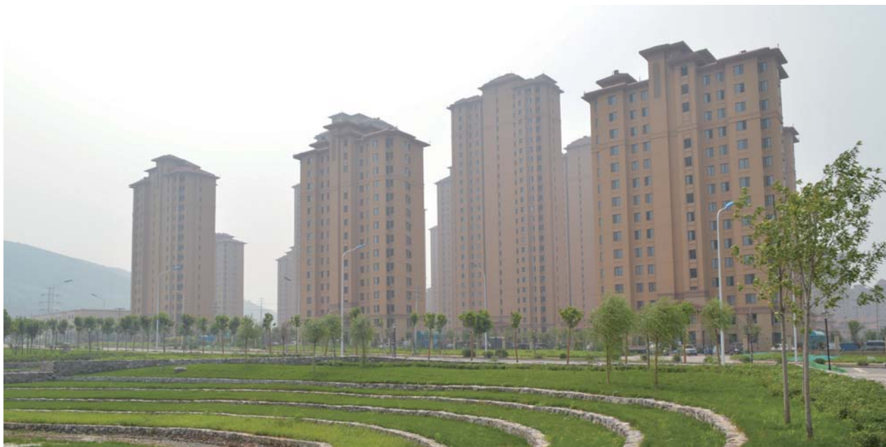
Construction projects in demonstration small town supported by Jizhou Sub-branch
