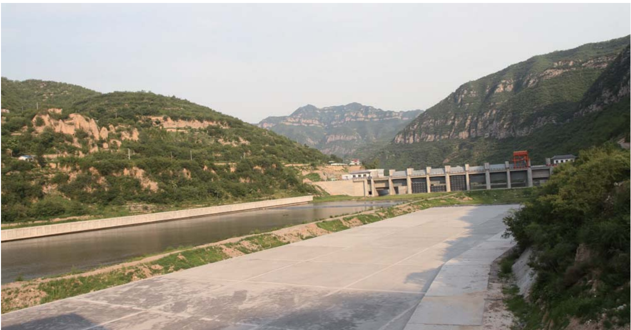
Xinanquan water supply renovation and expansion project supported by Shanxi Branch
