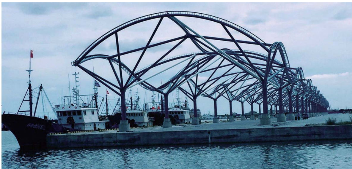
Support for Comprehensive Improvement Construction Project of Ancient Fishing Port in Lvzigang Town, Qidong by Nantong Branch
